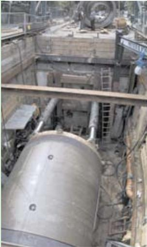
Normally, the pipe can be held horizontal while the jacking station is used to push home the joint. For the first few pipes, the lead pipe may have to be restrained until sufficient weight is available to resist the movement while trailing pipe is joined. Pre-cast lifting anchors are available for most pipe diameters to ensure proper and safe handling practices.
